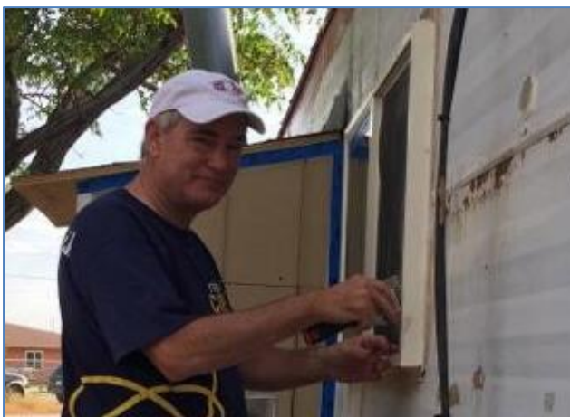
Joel Hendryx, M.D., Chief Medical Officer, scrapes old paint from a window frame before hitting it with a fresh coat.
