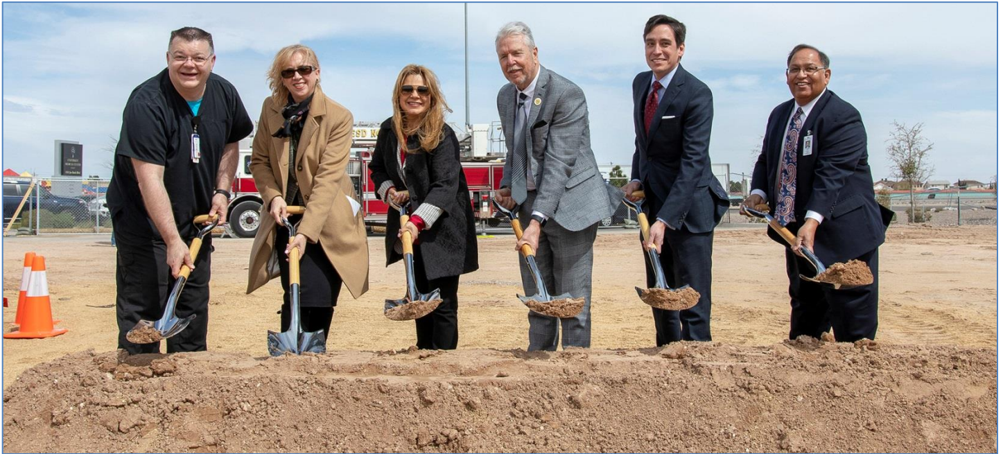
UMC and community leaders get our new East Emergency Department started at the March 15 groundbreaking ceremony in a lot next to the UMC East Clinic. From left, Eric Johansen, Emergency Department Director; Maria Zampini, UMC Chief Operating Officer; Joy Martinez, UMC Board of Managers; County Judge Ricardo Samaniego; County Commissioner Vince Perez; and Jacob Cintron, UMC President & CEO.
